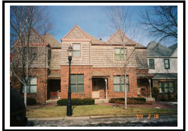
Photo 10 - 34 Yr. Old Apartment (56 Units)
