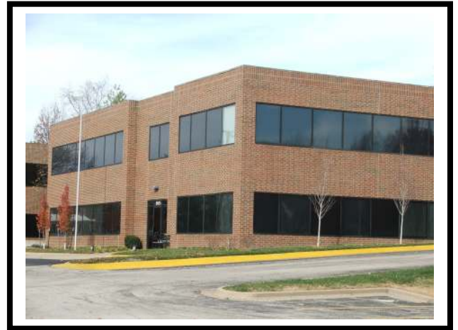
Photo 22 - 31 Yr Old Office Building
