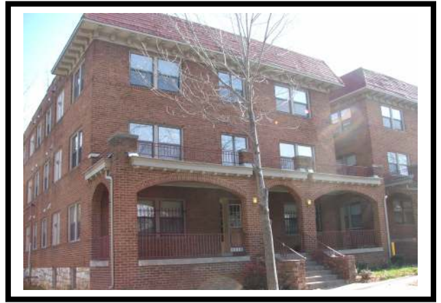
Photo 14 - 79 Yr. Old Apt Bldg (18 Units)
