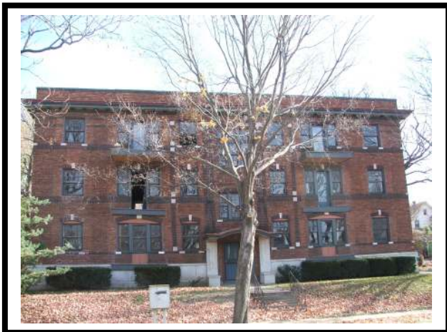
Photo 23 - 68 Yr. Old Office Renovation
